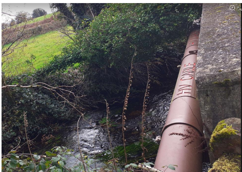
Figure 14 - 33kV network strapped to the side of this bridge across Caha River.
