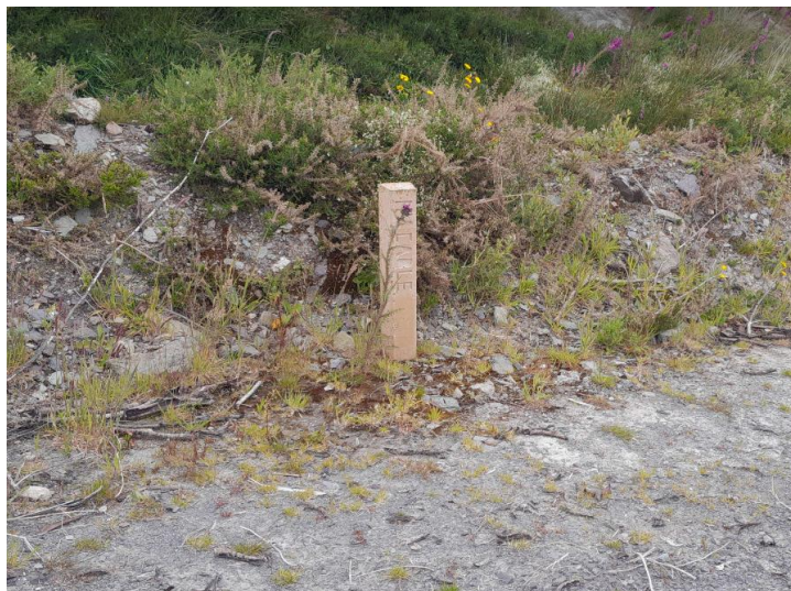
Figure 17 - WTG Radial cable markers
